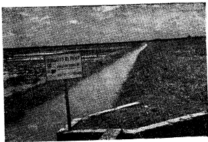
Main canal and a check gate for a 16-inch pump in Boyaninuan, La Paz, Tarlac.
